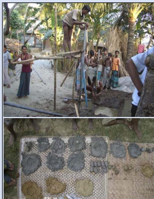
**Figure 4. Community initiative of the local driller for targeting safe sediments for tubewell installation in Bangladesh – the emergence of “the sediment colour concept”.**
